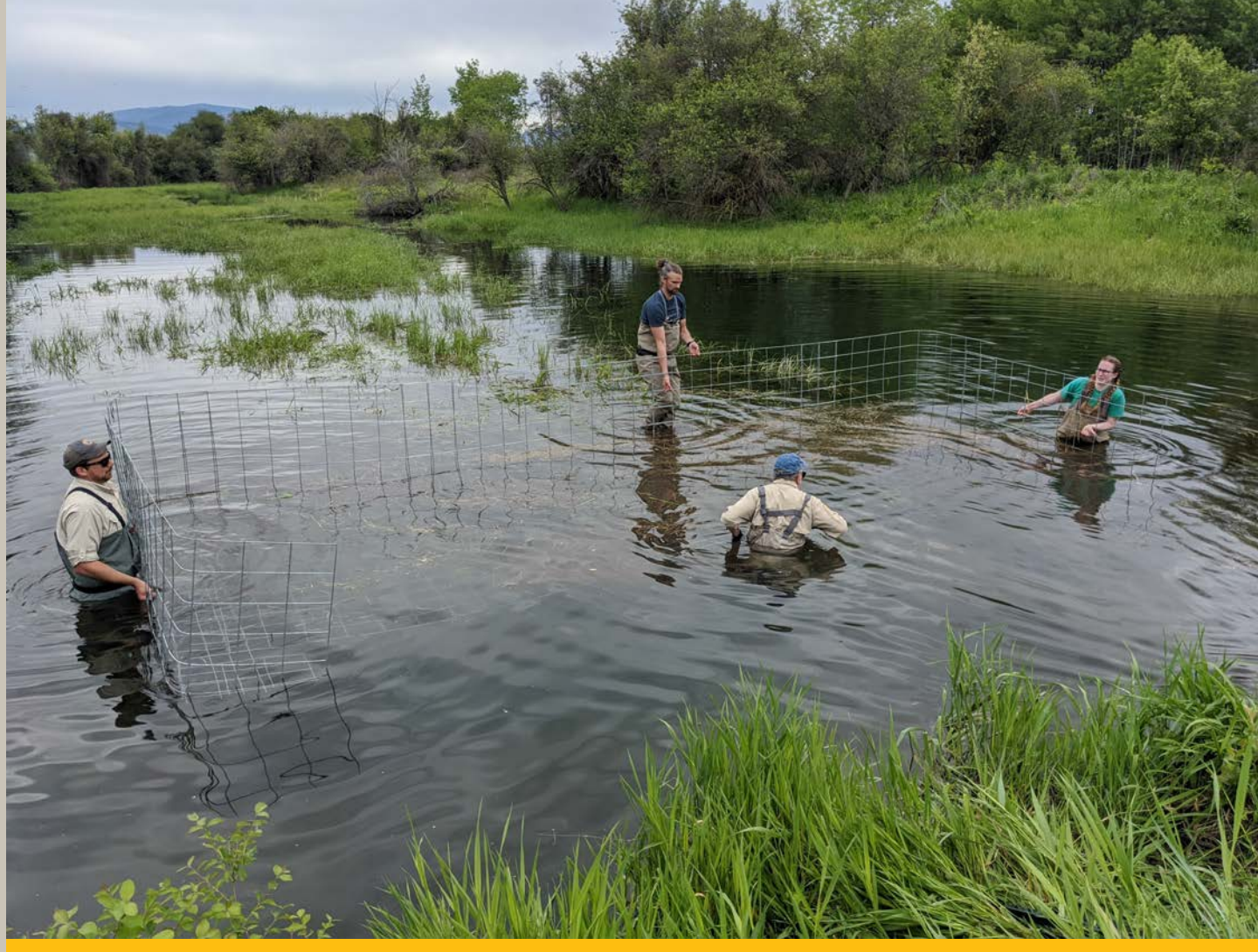
Montana Beaver Conflict Mitigation Project team members install double-culvert exclusion device at Council Grove State Park, with hands-on support from MT Fish, Wildlife & Parks (photo by Sarah Bates).
